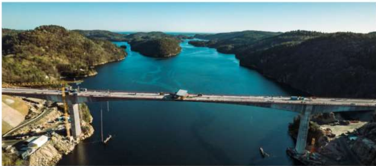
Figure 1: Trysfjordbrua bridge under construction (Photo: Amit Verma – Ribe betong).
